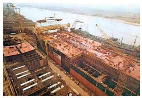
Assembly of a super tanker in the building dock.
