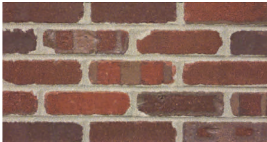
Standard 3/8" Mortar Joint
