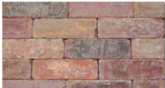
No Mortar Joint (Dry-Stacked)
