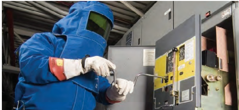
Figure 3 - check of covers, doors and all bolts
