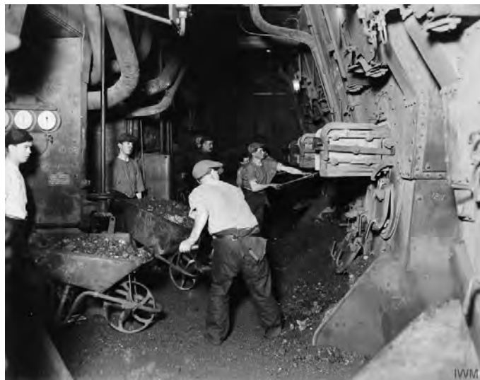
Steam ships boiler room
