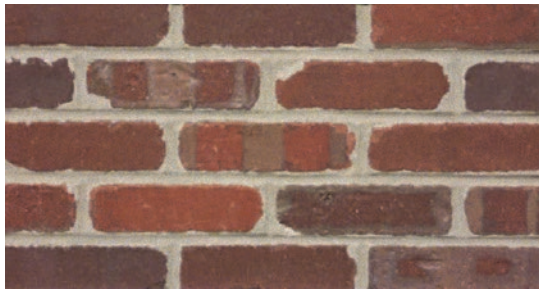
Standard 3/8" Mortar Joint
