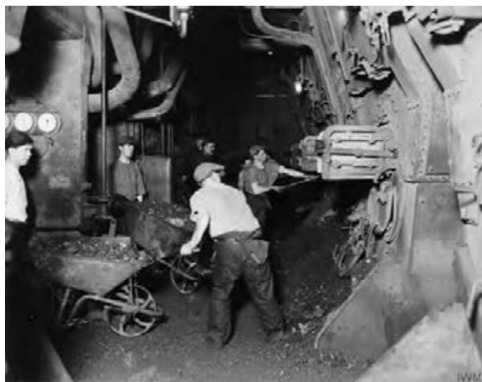
Steam ships boiler room
