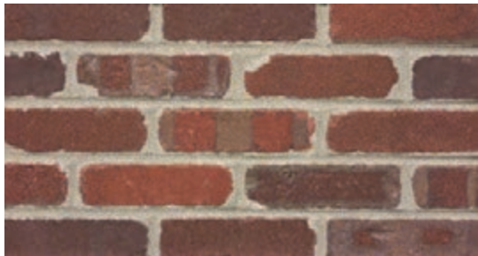
Standard 3/8" Mortar Joint
