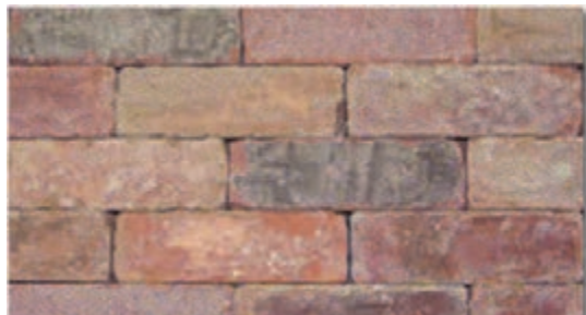
No Mortar Joint (Dry-Stacked)
