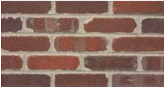
Standard 3/8" Mortar Joint
