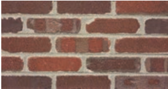
Standard 3/8" Mortar Joint
