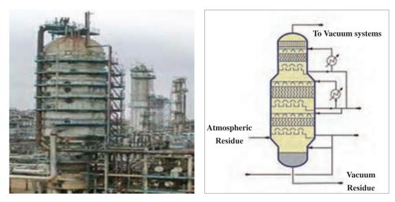
Fig. 20: Vacuum distillation tower
